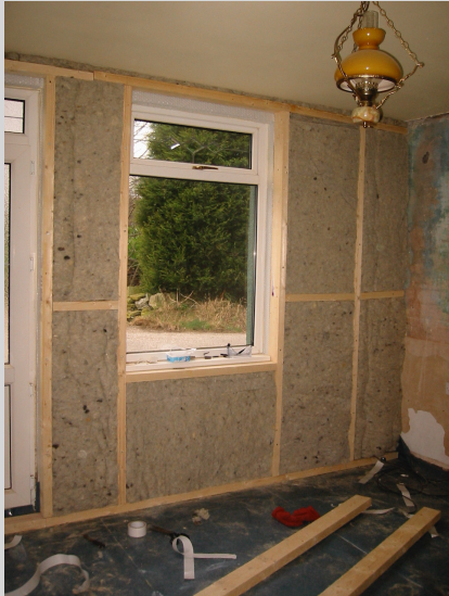
Sheeps wool internal wall insulation.
