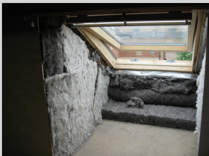
Sheeps wool insulation in the loft.
