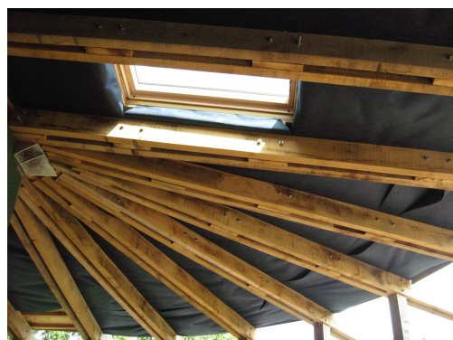
Internal view of completed rafters with roofing felt and skylight above.
